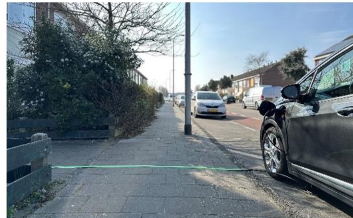
Platte kabel (bron: FlatPower) 1
